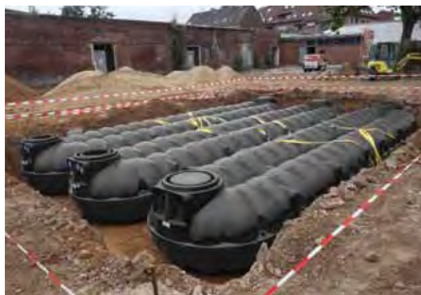
Installation NEO buffertank 3 x 20 000 l
