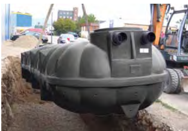
Installation NEO infiltrationstank 10 000 l
